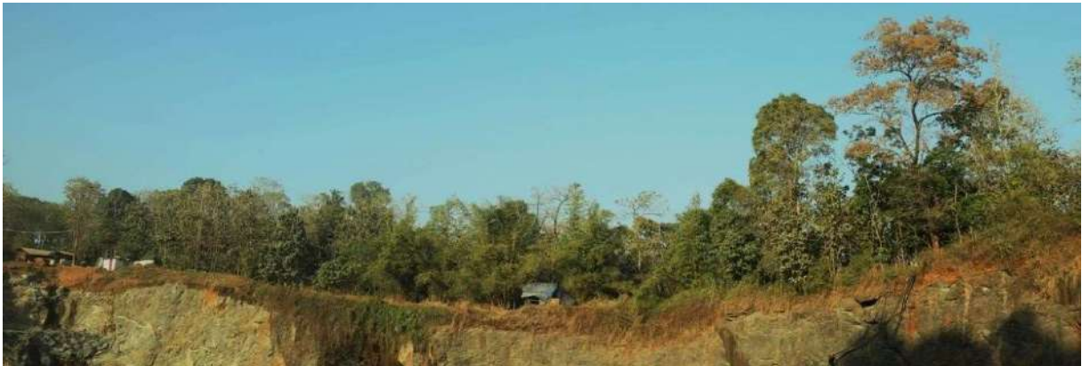
Green Belt to reduce Noise Pollution
